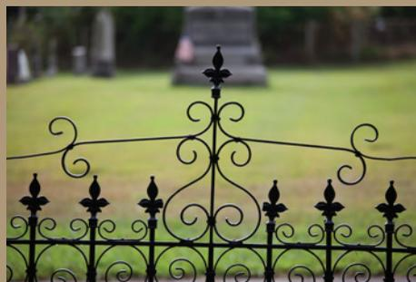
**TECHNICAL DETAILS:** In this restoration project the fencing had been disassembled and stacked in piles behind the church. The wrought iron fence was rusted and bent and the posts were missing. Shrock restored the pickets and reconstructed the posts using a photo of the post finials. By installing the fence further back from the new sidewalk, damage during snow clearing is prevented.
