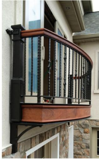
With the remodel of the master bedroom suite, these homeowners added an aluminum balcony structure with forged aluminum balusters and large posts made of marine grade cast aluminum. The structure of the balcony extends inside and is fastened to the existing joists of the house. This gives additional strength and security.
