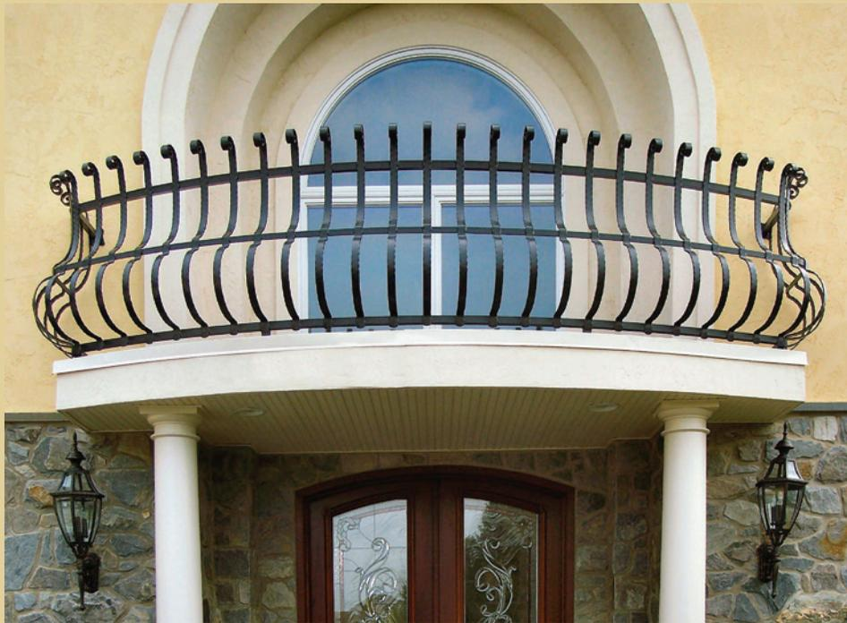
For this Mediterranean-style home, belly railings are used to accent the balcony and windows. They provide a striking contrast to the stucco and stonework of the exterior walls.
