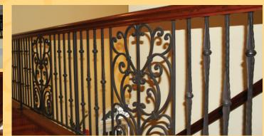
There is a metal subframe for the cherry top rail, which is fastened with countersunk screws that are invisible from the side. The bottom rail keeps the panels and balusters in place and is two inches above the steps. This project was a complete metal package.
