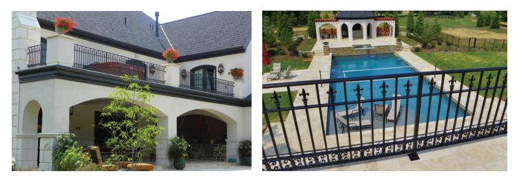
This 10,000-square-foot house has a large balcony with long stretches between stucco pillars. The aluminum balcony railing was designed using four horizontal rails to bridge the distance between the columns, plus two posts were placed in each railing section to give additional support. The railing has solid pickets and a cap and channel top rail.
