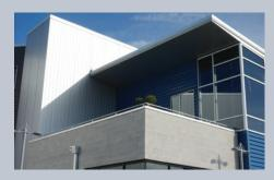
In order to bring the exterior walls to code height on the terrace, a top rail was needed. Since the terrace is open to employees for their breaks during pleasant weather, the choice was to use metal railing that did not obstruct the view. The terrace wall is topped by an anodized aluminum miniature two-rail system. The railing adds to the clean lines of the building.
