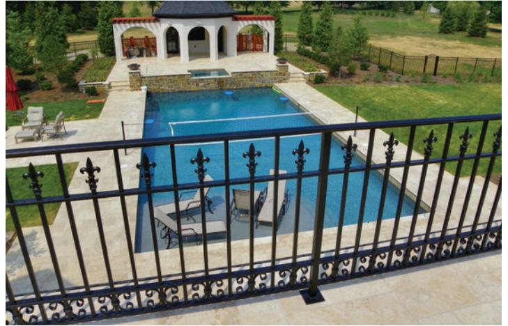
This 10,000-square-foot house has a large balcony with long stretches between stucco pillars. The aluminum balcony railing was designed using four horizontal rails to bridge the distance between the columns, plus two posts were placed in each railing section to give additional support. The railing has solid pickets and a cap and channel top rail.
