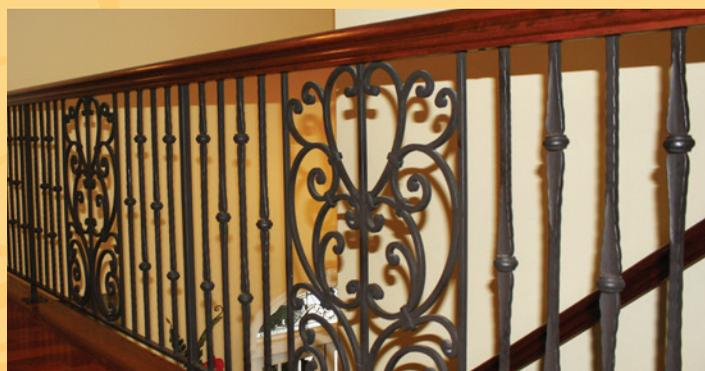
**TECHNICAL DETAILS:** The panel design is Tuscan Style Railing with vertical forged steel balusters. The balusters have alternating knuckles; one near the top and one near the bottom. The flat black powder coating is accented by subtle antique gold sprinkles and the railing has a lightly hammered finish.
