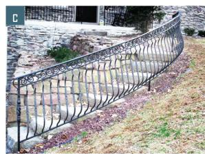
Basically there are five different belly railing profiles to choose from. Combining those with multiple materials gives many options. It is possible to have smooth, hammered, flat bar, or square pickets. The pickets can be twisted, as well as bellied. The top of the belly picket can have a top curl, a frieze, or a straight handrail.
