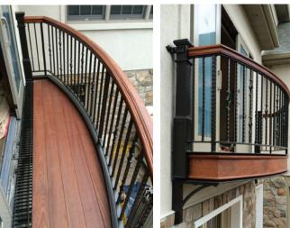
With the remodel of the master bedroom suite, these homeowners added an aluminum balcony structure with forged aluminum balusters and large posts made of marine grade cast aluminum. The structure of the balcony extends inside and is fastened to the existing joists of the house. This gives additional strength and security.
