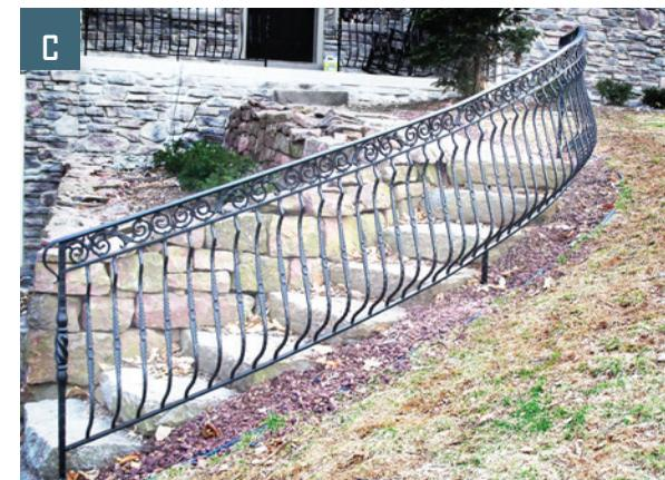
Basically there are five different belly railing profiles to choose from. Combining those with multiple materials gives many options. It is possible to have smooth, hammered, flat bar, or square pickets. The pickets can be twisted, as well as belled. The top of the belly picket can have a top curl, a frieze, or a straight handrail.
