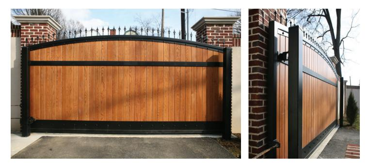
▲ This rear courtyard sliding gate is built for maximum security. It is made of 2 ½" thick, custom milled white oak and weighs over 3,000 pounds. There are security posts on the side of the gate.
