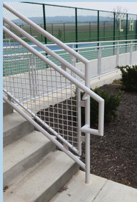
◀ Components of the stairway railings are custom woven wire mesh panels and hot-dip galvanized steel pipe railing, which is powder coated gray.
