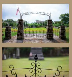
TECHNICAL DETAILS: In this restoration project the fencing had been disassembled and stacked in piles behind the church. The wrought iron fence was rusted and bent and the posts were missing. Shrock restored the pickets and reconstructed the posts using a photo of the post finials. By installing the fence further back from the new sidewalk, damage during snow clearing is prevented.
