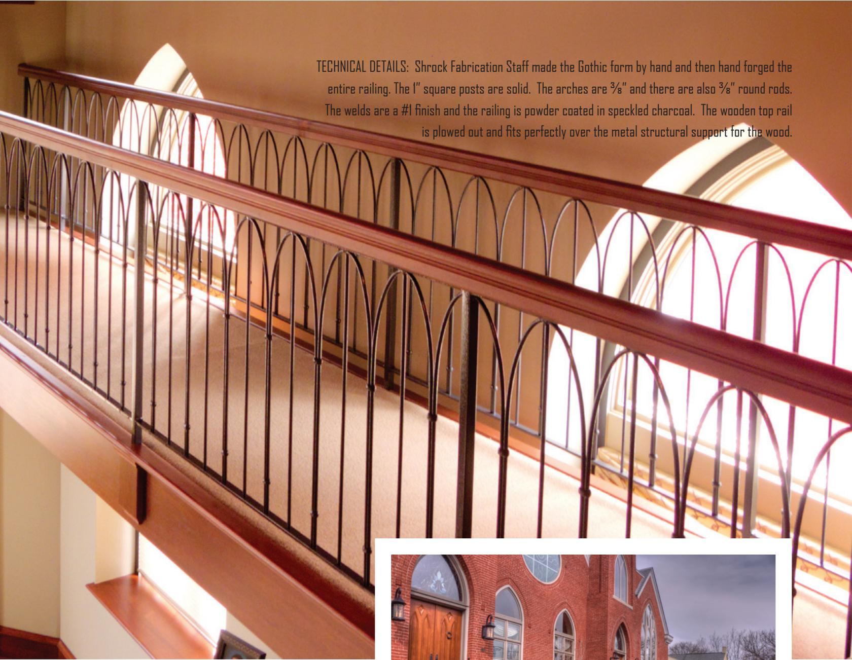
TECHNICAL DETAILS: Shrock Fabrication Staff made the Gothic form by hand and then hand forged the entire railing. The 1" square posts are solid. The arches are  $\frac{3}{8}$ " and there are also  $\frac{3}{8}$ " round rods. The welds are a #1 finish and the railing is powder coated in speckled charcoal. The wooden top rail is plowed out and fits perfectly over the metal structural support for the wood.
