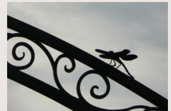
TECHNICAL DETAILS: A freelance artist was able to hand draw the scrollwork for the arch, which was traced with CAD. The two crosses with sharpened edges and the intricate dragonflies with details on the wings and tail were hand forged out of steel. The archway, of all solid steel bar, is 177" wide and has a clearance of 10'3". It was hot-dip galvanized and painted with European wrought iron paint.
