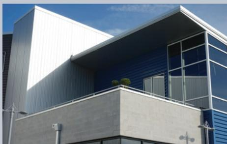
In order to bring the exterior walls to code height on the terrace, a top rail was needed. Since the terrace is open to employees for their breaks during pleasant weather, the choice was to use metal railing that did not obstruct the view. The terrace wall is topped by an anodized aluminum miniature two-rail system. The railing adds to the clean lines of the building.
